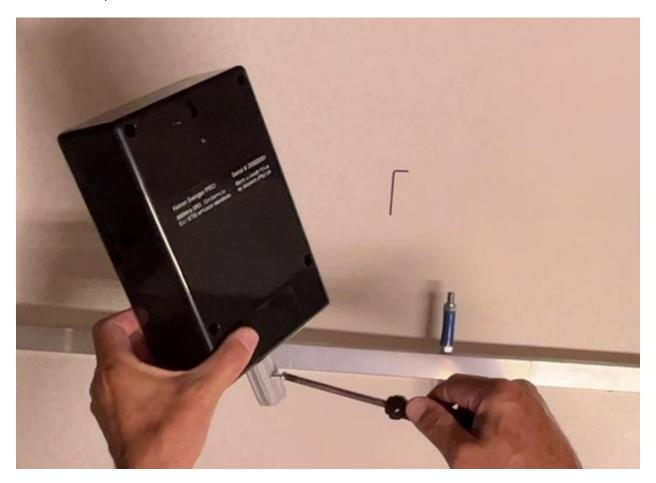
Push the target into the top of the swinger arm so that "B" meets "B".
